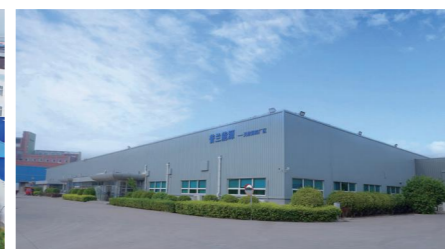
普蓝储能 PULAN ENERGY STORAGE 年产 AnnualCapacity : 3GWh
